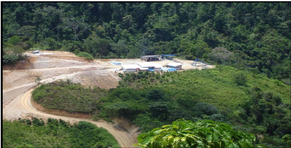
Plate 1: View of mine services area showing headframe and mine services area.
